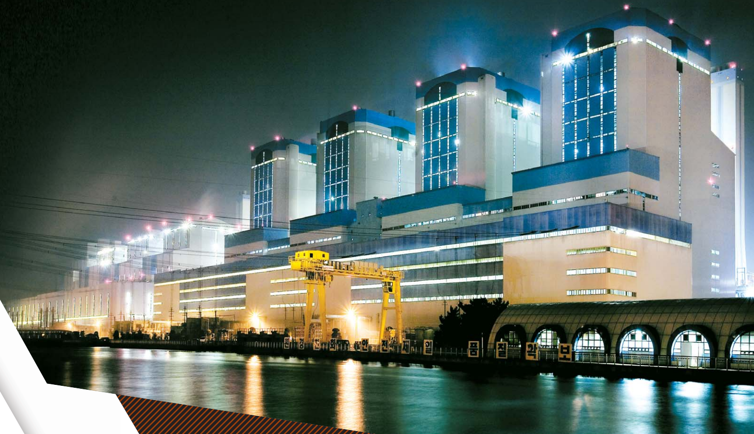
Dangjin Coal-Fired Power Plant(Unit 7 & 8)
